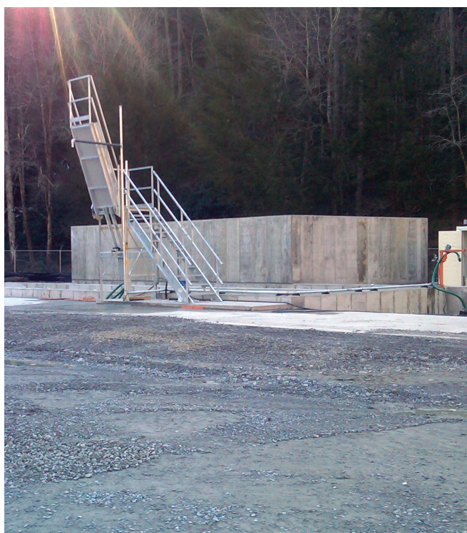
Above: New washout sump/water recycling system installed at our Wyoming Co., WV ready mix concrete plant.
